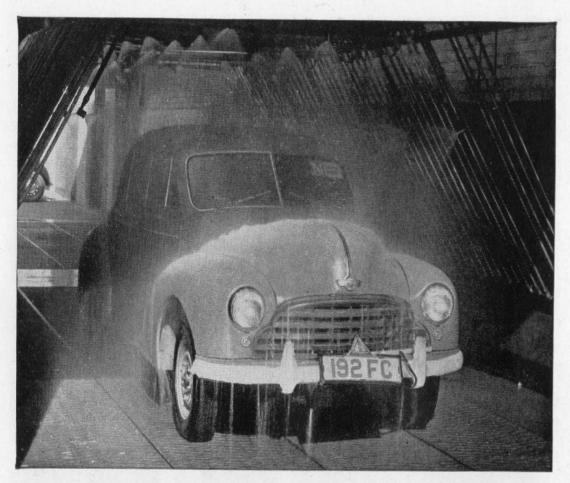
MAKING SURE, and very sure indeed, that the car will withstand tropical rain is the reason for this cascade. Equalling a rainfall of fifteen inches an hour, fifteen hundred jets of water are directed on the car from all angles. Such a downpour quickly searches out the smallest chink in the assembly of the bodywork.
